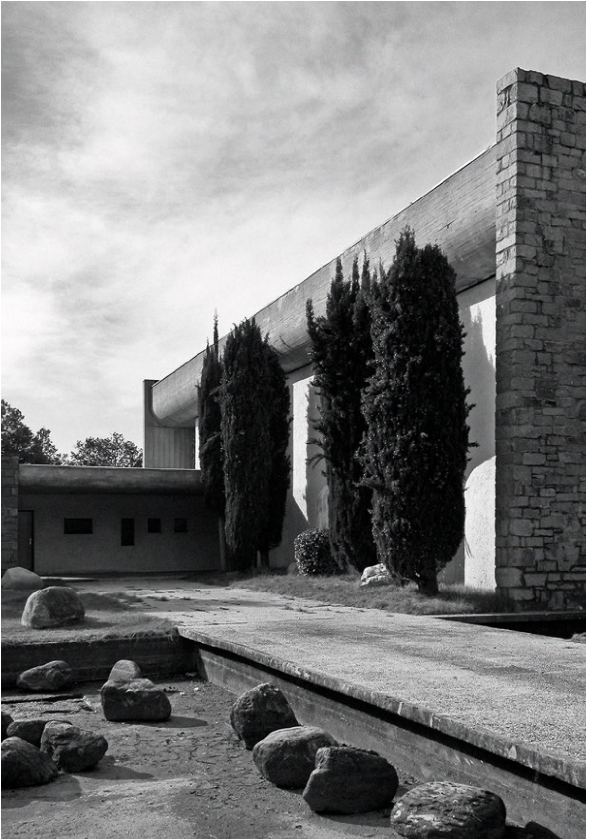
Headquarters, Parc de Belloch, Barcelona
